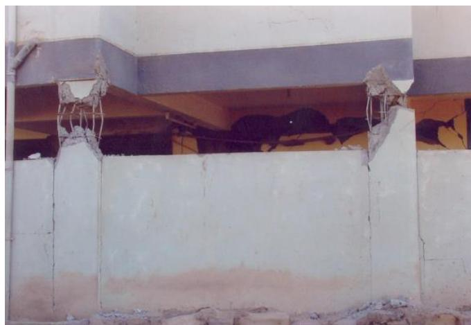
*Figure 4. Earthquake-damaged short columns.*
